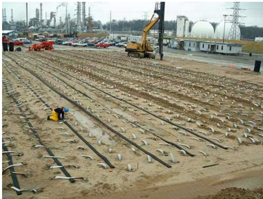
Gambar 1 : Pemasangan Prefabricated Vertical Drain (PVD)
